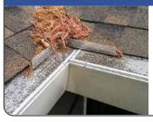
Roof valleys can cause excessive rain water and debris build up creating challenges for all gutter guards. Rainwater diverters help hold debris back and away from the gutter guard.
